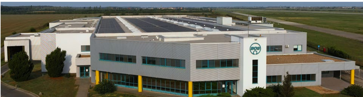
BOS Plant Arad with Photovoltaic Panels installed in 2025
